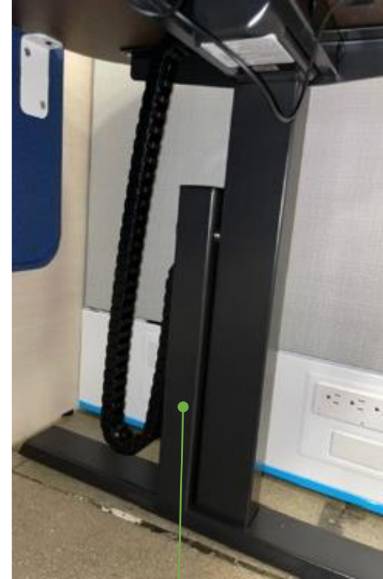
VERTICAL WIRE MANAGERS ATTACHED TO HATS IN EACH STATION
